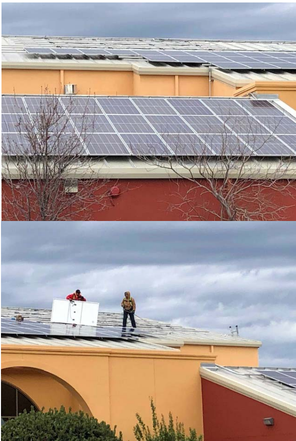
The Roof Of the Life Center
